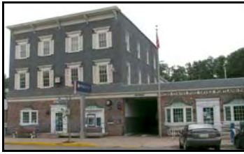
PNC Bank and Post Office
