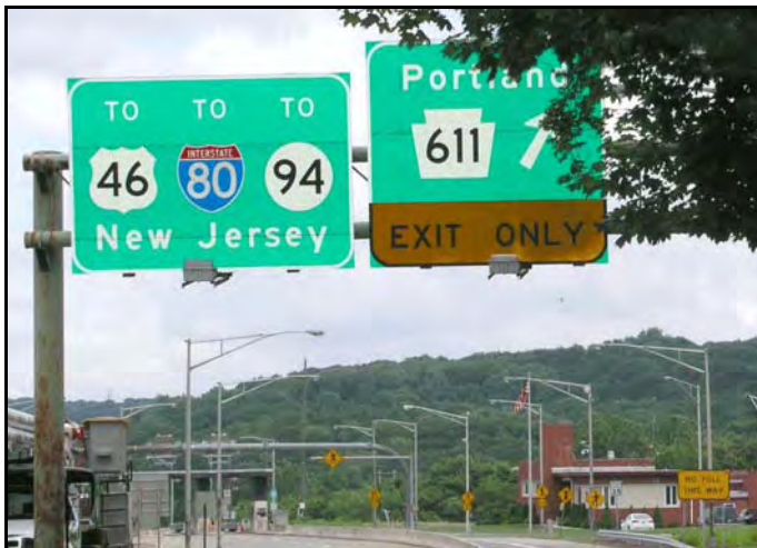
Route 611 (arterial) Approaching Bridge to Columbia, NJ
