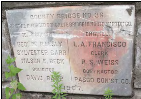
Route 611/Jacoby Creek Bridge
