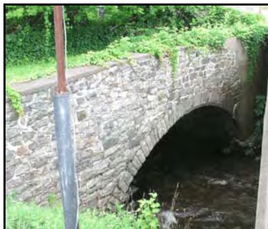
Stone Arch Bridge
